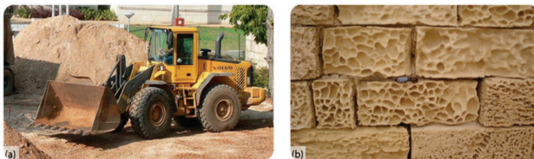
Figure 4. (a) Human activities are responsible for enormous amounts of mechanical weathering, by digging or blasting into rock to build homes, roads, subways, or to quarry stone. (b) Salt weathering of building stone on the island of Gozo, Malta
