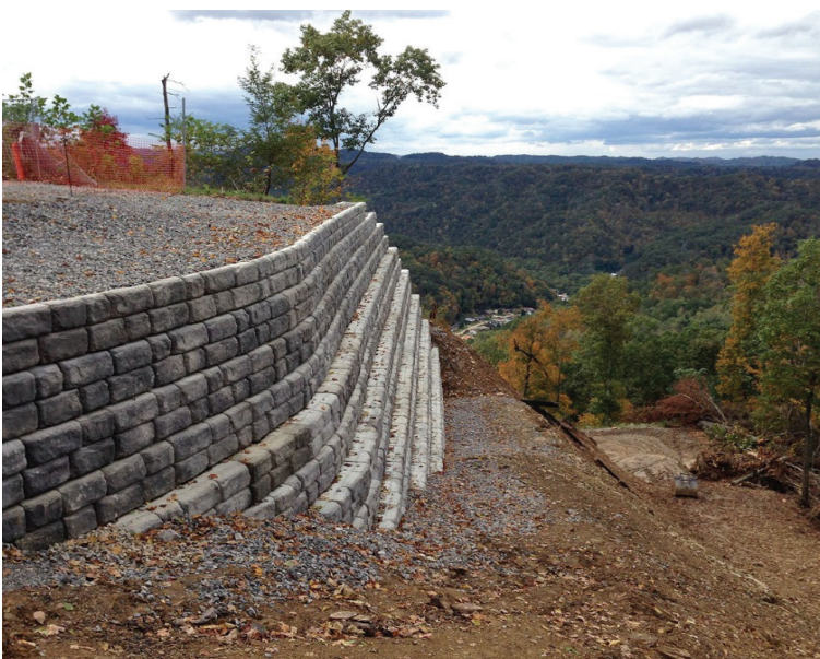
Figure 12. Retaining wall to stabilise a slope.
